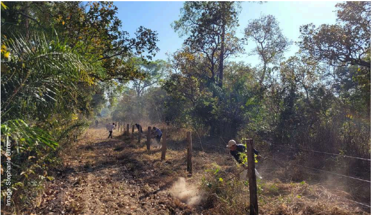
Construction of firebreaks on Indigenous Land. A firebreak is a strategically cleared strip of land created to prevent the spread of fires. This technique involves removing or reducing combustible material (such as leaves, dry branches, and grass) from a specific area forming a physical barrier that hinders or blocks the advance of flames.
