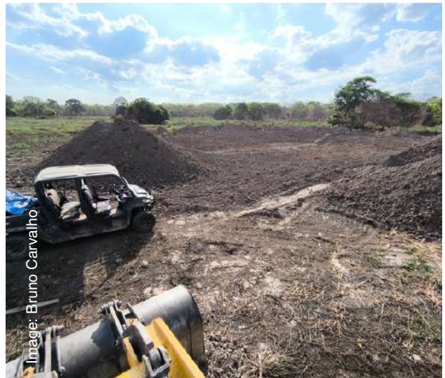
Construction of ponds in the São Francisco do Perigara Reserve to provide hydration for animals affected by the fires and during future droughts.
