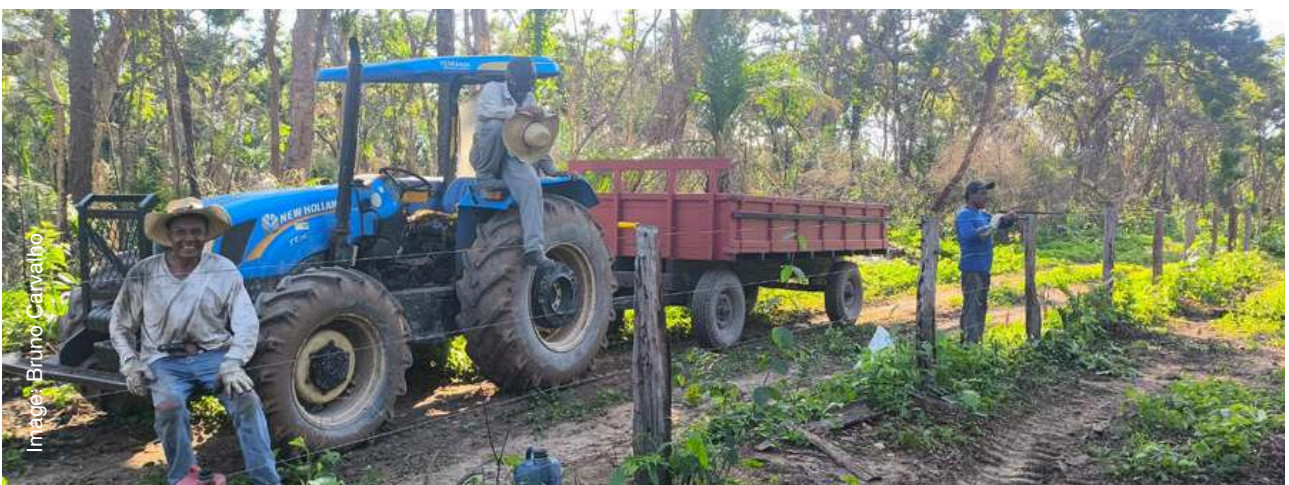
Installation of new fences throughout the property.
